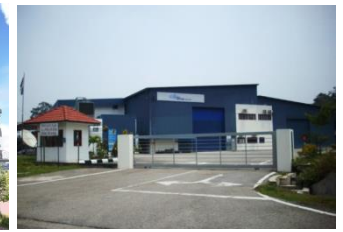
Plant expansion, Bentong
